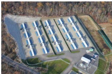
20 MW, 5 MWh Flywheel plant
