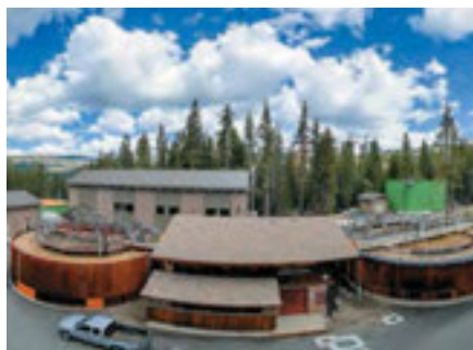
Above: The Donner Summit Wastewater Treatment Plant, designed by Stantec, uses tertiary treatment with membrane bioreactors to filter and treat wastewater discharged into the South Yuba River. Below: The Silicon Valley Advanced Water Purification Center, located in northern San José, uses microfiltration, reverse osmosis and ultraviolet light to purify wastewater for industrial and agricultural uses.
