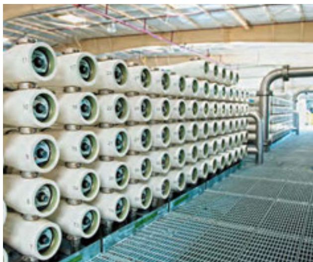
Above: The Donner Summit Wastewater Treatment Plant, designed by Stantec, uses tertiary treatment with membrane bioreactors to filter and treat wastewater discharged into the South Yuba River. Below: The Silicon Valley Advanced Water Purification Center, located in northern San José, uses microfiltration, reverse osmosis and ultraviolet light to purify wastewater for industrial and agricultural uses.
