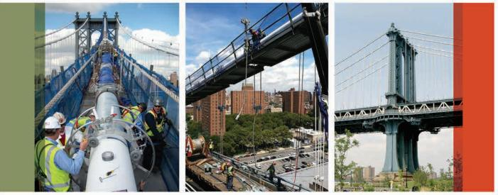
With 80 years of service, the Manhattan Bridge suspenders were deteriorated and due for replacement. All 1,256 suspender ropes were replaced, with some key modifications.
