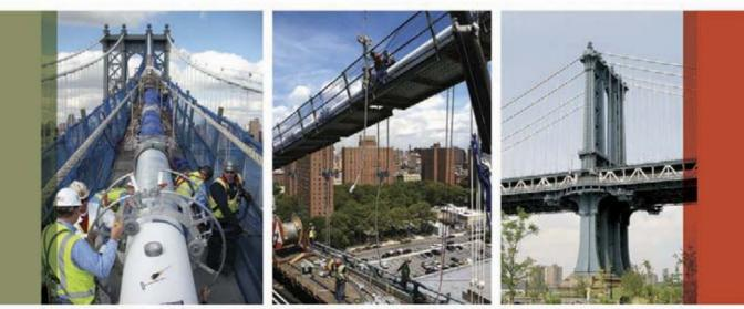
With 80 years of service, the Manhattan Bridge suspenders were deteriorated and due for replacement. All 1,256 suspender ropes were replaced, with some key modifications.
