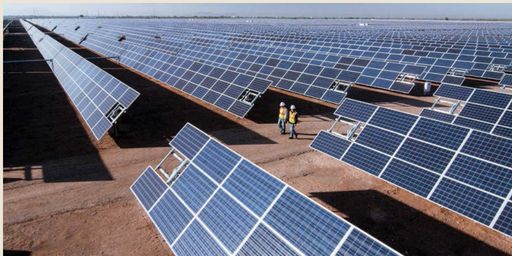
Black & Veatch provided engineering, procurement and construction services for Arizona Public Service's Solana Generating Station in Gila Bend. The solar power plant sits on 400 acres and produces 32 megawatts of electricity—enough capacity to power 8,000 homes and businesses.
