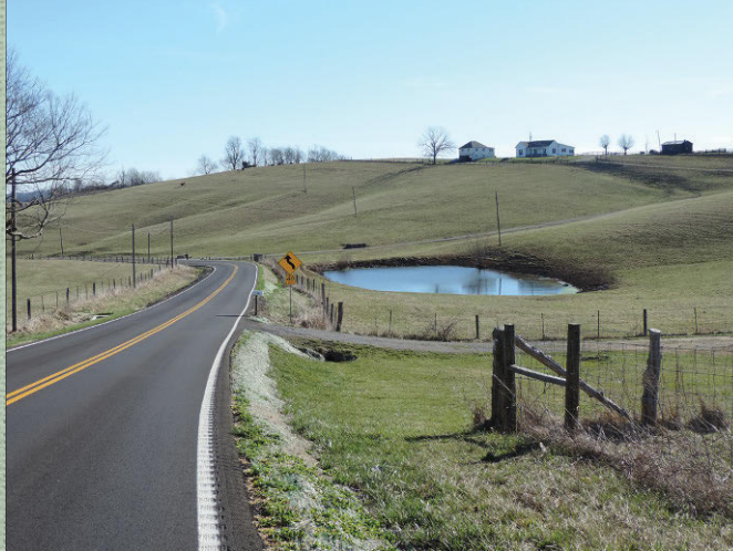
The EA Partners plan widened KY 1194 to 20 total feet throughout the 6.6-mile route, added a fresh coat of asphalt, bright striping, signage and rumble strips to improve the safety of the roadway. Since completion, there have not been any injury crashes along the route.
